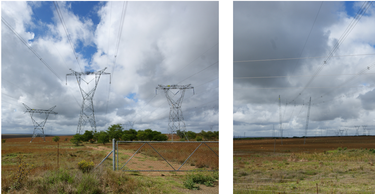
Figure 10: Examples of the 517E and 517F towers to be erected as part of the Juno-Gromis powerline (left). Example of the 529A cross-rope suspension tower (right).
